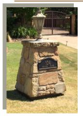
Material: Monument Base is to be constructed of masonry material. Masonry material is to match exterior of home (stone/rock/stucco/etc.) Masonry Light Monument is to be 43" in height from grade. Masonry Light Monument base is to be 31" square Masonry Light Monument top is to be 22 ½" square Masonry Light Monument cap is to be 4" thick with a 2" overhang on 4 sides.
